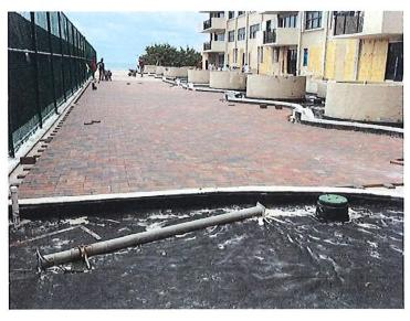
The expansion joint in the planter in the east south corner was installed, Blue coast waterproof the area and it is going to have the pavers so we will open the stairs for the tennis players
