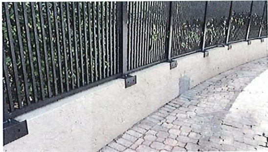
The fence company is welding the plates by C pool
